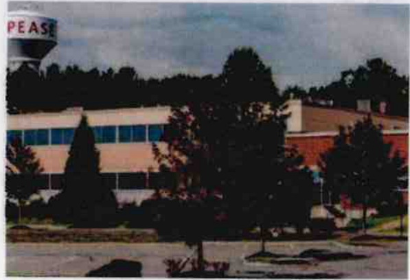
Teledyne Instruments, Inc. 162 Corporate Drive - Portsmouth, NH 102,400 SF
