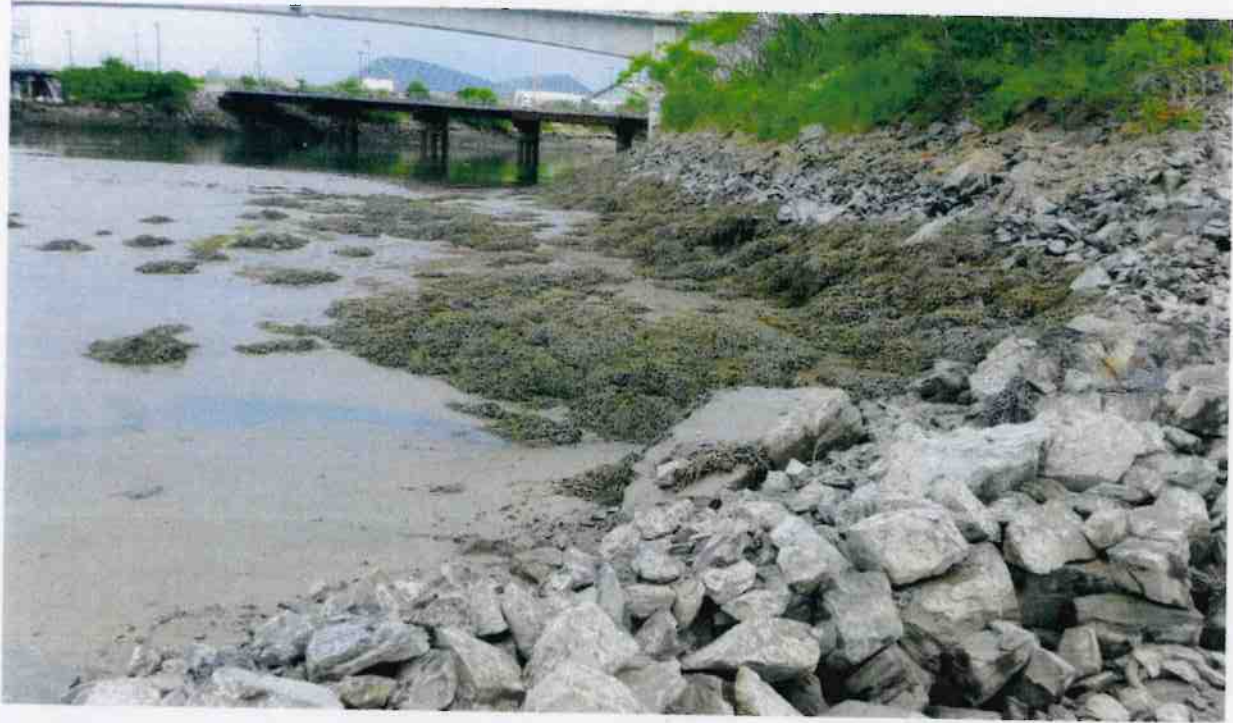
Existing Armored bank
